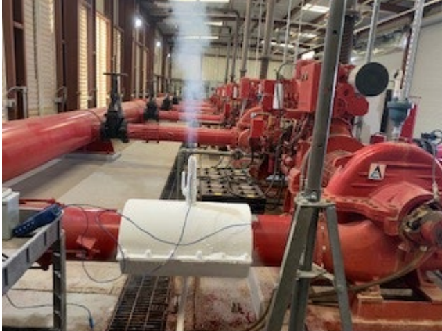
Pipe Freeze in progress
